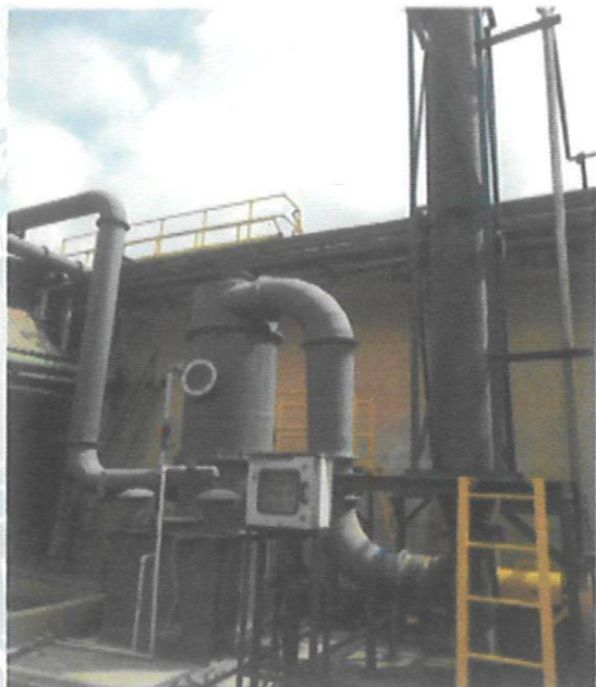
Scrubber System in ETP and Odour Monitoring System
