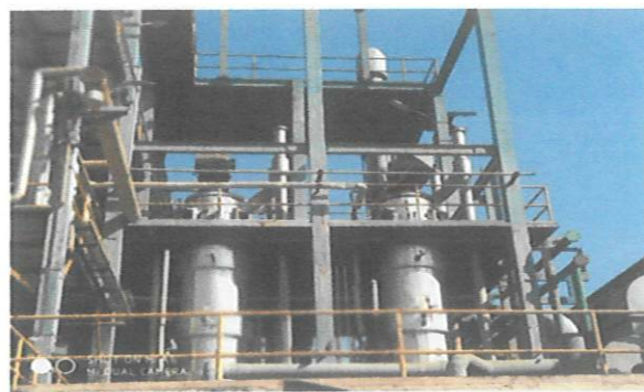
Vertical Thin Film Dryer (VTFD)
