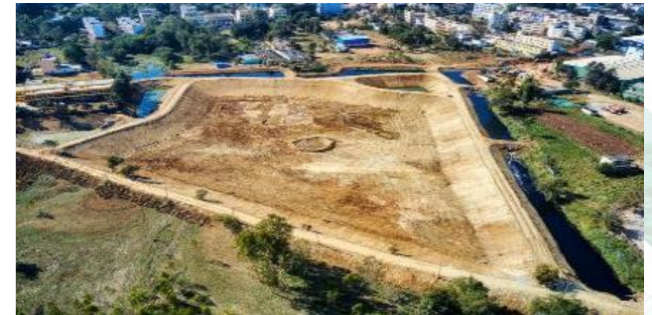
Yarandahalli Lake Revival: 95% of Phase-I rejuvenation work completed
