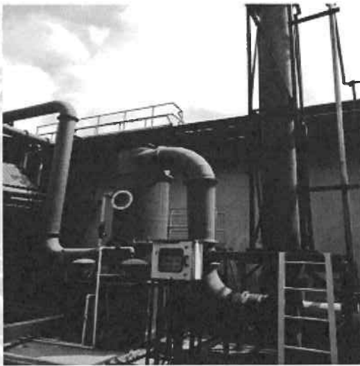
Scrubber System in ETP and Odour Monitoring System
